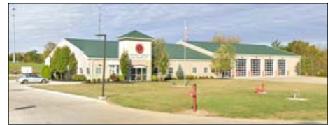
Concord Township Fire Station
